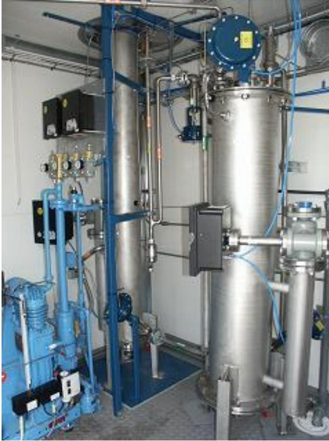
**Figure 7.** Biogas upgrading unit (water scrubber) at Plönninge biogas plant, Sweden. (Source: Courtesy: BioRega, Sweden; Peter Karlsson, Biogas Öst seminarium 2011-04-01)
